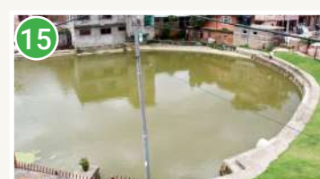
15. Po Pukhu: Recently renovated, this pond receives water from Rajkulo, the irrigation canal that serves the area. The pond helps to recharge the ground to feed to the wells.
