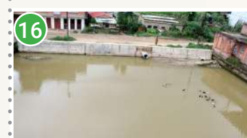
16. Na Pukhu: This pond receives water from the Rajkulo irrigation canal along with storm water and protects the area from landslide. The pond is also used for several rituals.
